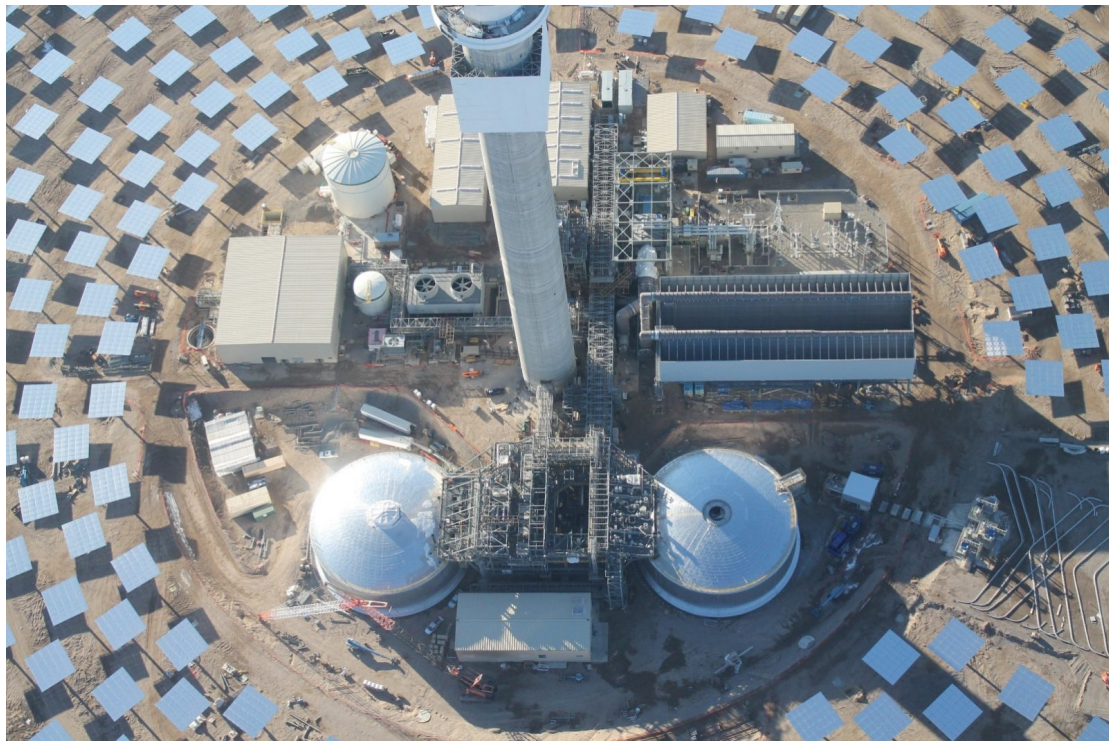
Figure 11 Crescent Dunes (Nevada) CSP plant picture.
